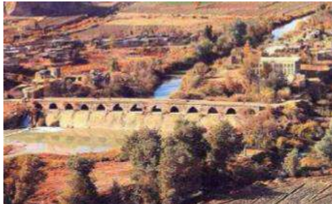
Figure 5. Amir dam in Iran (courtesy ICOLD, 2007)
