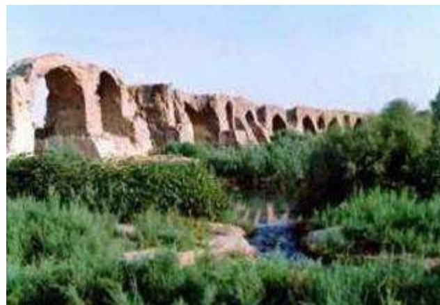
Figure 4. Shadorvan dam-bridge in Iran (courtesy, ICOLD, 2007).
