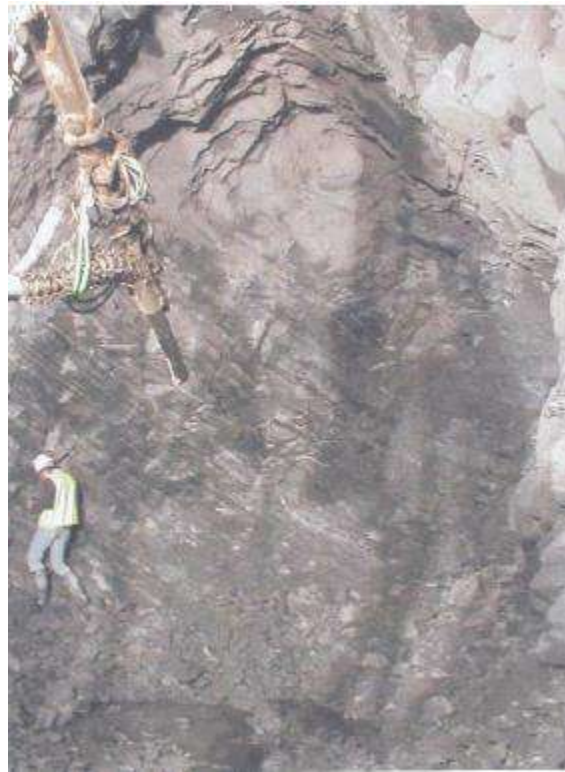
Figure 2. Application of sprayed concrete in Odelouca tunnel
