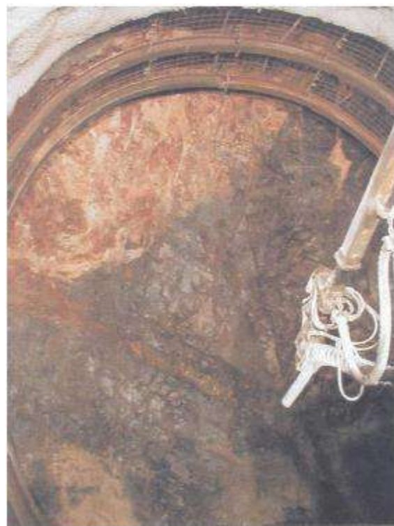
Figure 3. View of Odelouca tunnel with steel ribs
